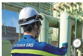
▲ Check meter scale from control room
